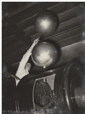
Construction of the enormous 1,000,000 volt X-ray tube in 1939. Images courtesy of St Bartholomew's Hospital Archives (Ref: RD/2/2/6)
